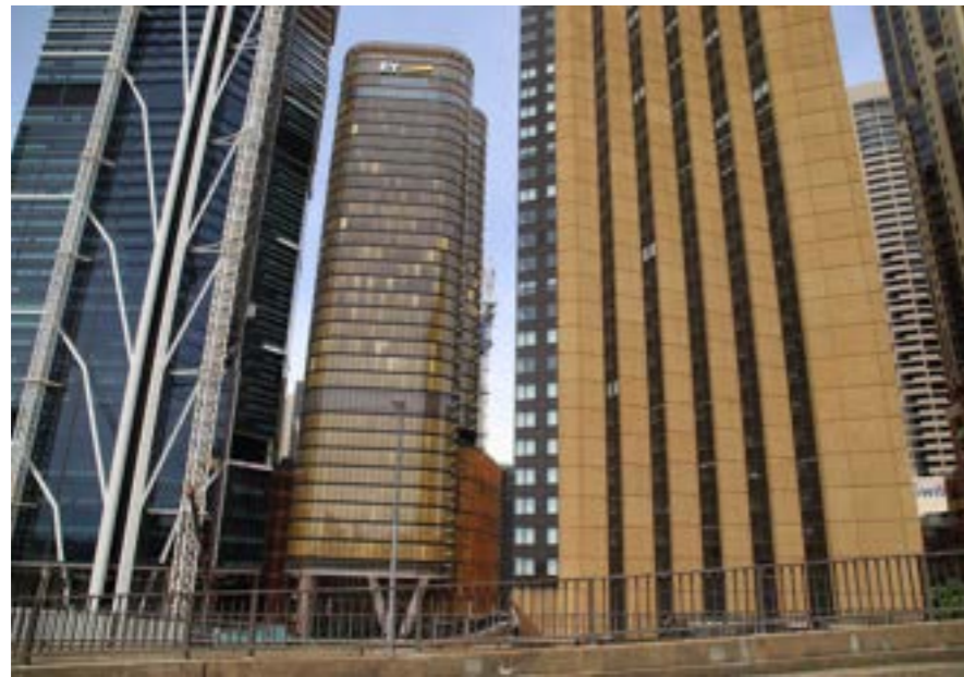
Plate. 3 View north to tower development adjacent to the southern side of the Cahill Expressway
