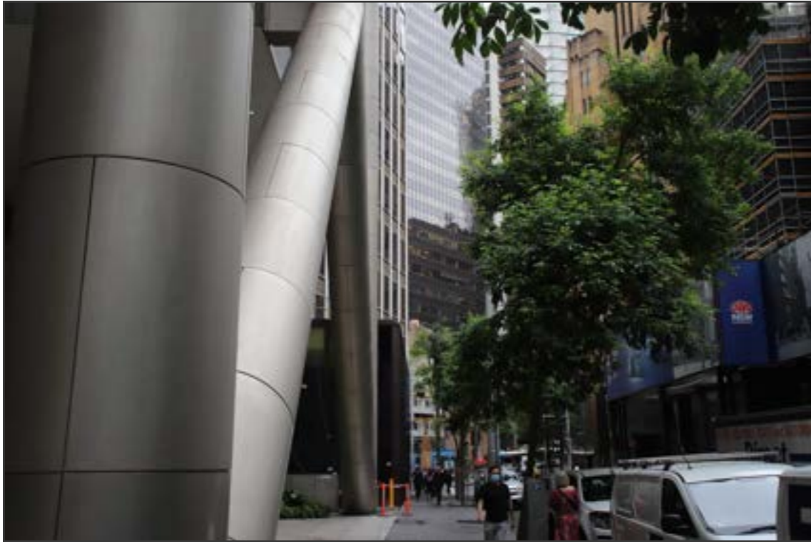
PHOTOGRAPH SHOWING CURRENT CONDITION
