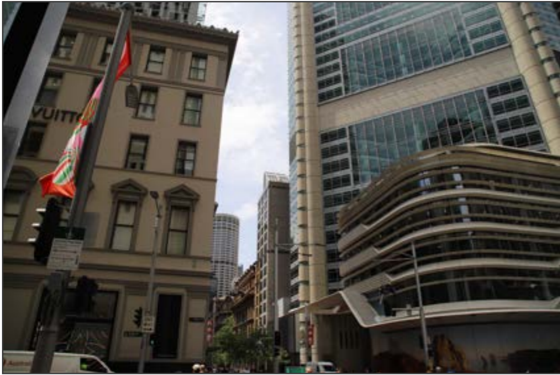
PHOTOGRAPH SHOWING CURRENT CONDITION
