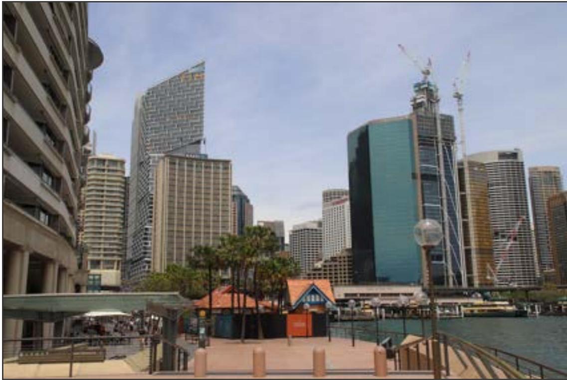
PHOTOGRAPH SHOWING CURRENT CONDITION
