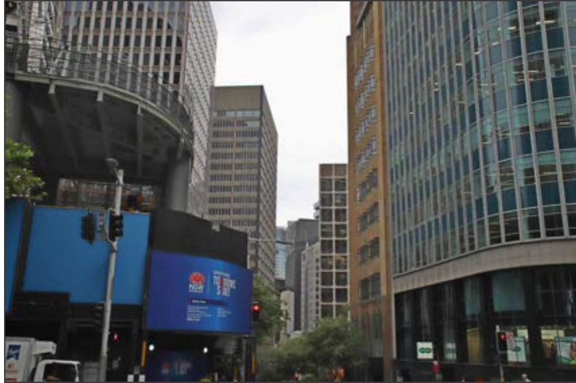
PHOTOGRAPH SHOWING CURRENT CONDITION
