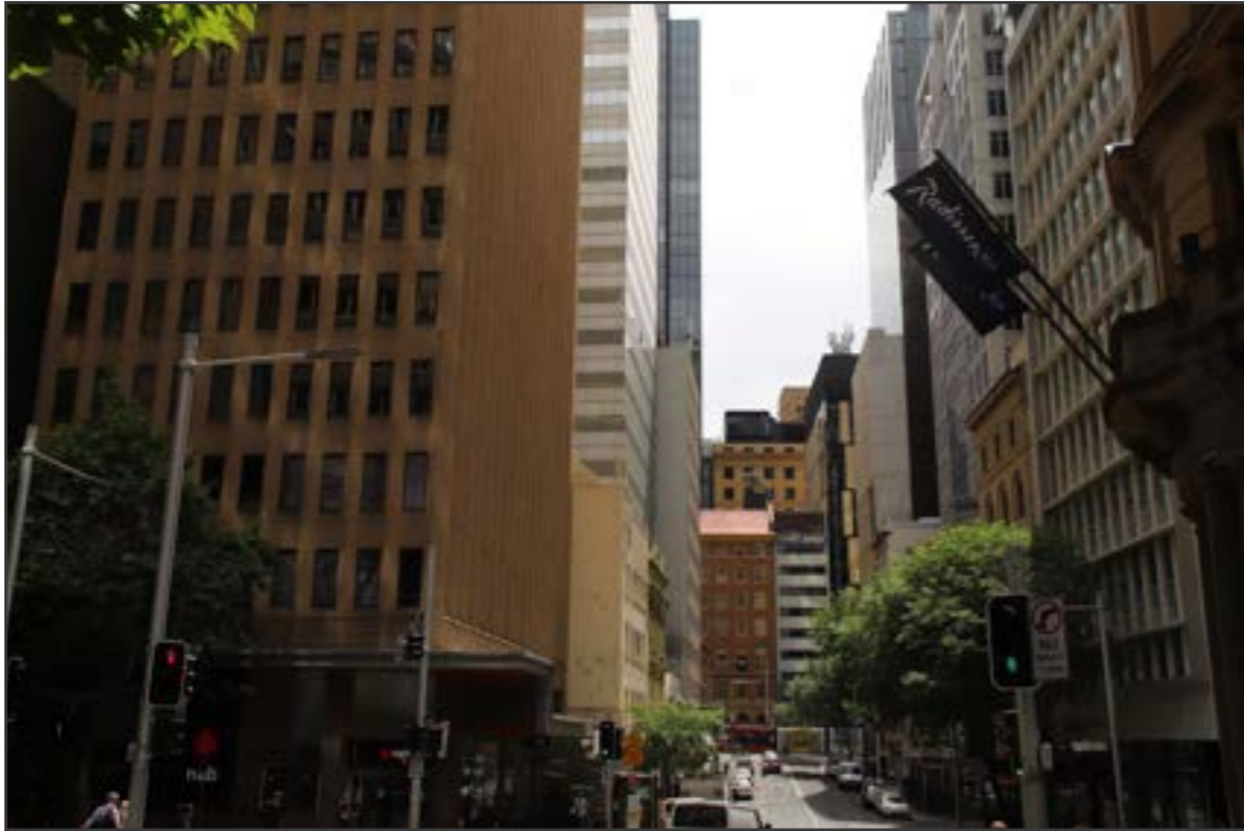
PHOTOGRAPH SHOWING CURRENT CONDITION
